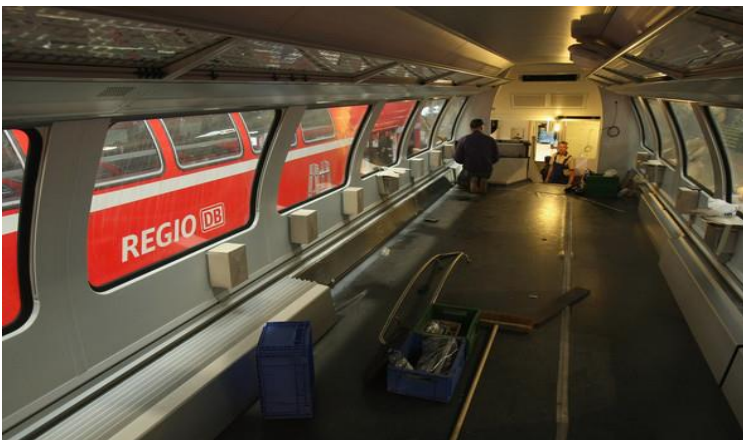
Internal Bonding (window surrounds, heating ducts floors, ceiling panels, light boxes)
