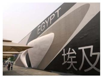
Curved sections of the Egypt pavilion at the China World Expo in Shanghai were made from a GRP laminate using heavily ATH filled Crestapol 1212 resin with Crystic LS30 ISO/NPG spray gelcoat, which met the stringent building fire regulations.
